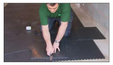
9 You can use an upside down tile as a cutting mat. Lay the tile down and align a metal rule with the marks you previously made.
