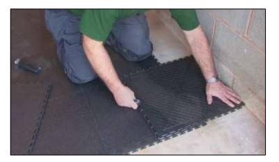
When a cut needs to be made, turn the tile upside down and push against the wall. Slide it slightly to one side to reveal the cut marker on the tile underneath.
