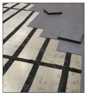
For an area of 5 metre x 7 metre =  $35m^2$ multiply the total area by 2.5 to work out how much conductive tubing is required.
