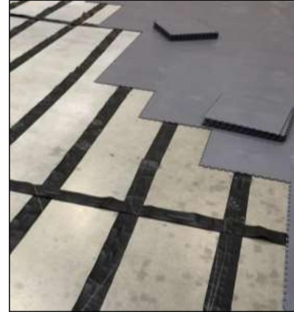
*For an area of 5 metre x 7 metre = 35m<sup>2</sup> multiply the total area by 2.5 to work out how much conductive tubing is required.*
