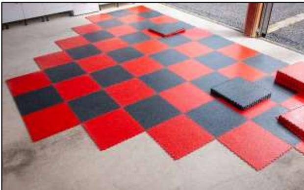
**5** Lay three rows of tiles on the chalk line along its whole length and gently tap into position so that it is exactly on the chalk line.
