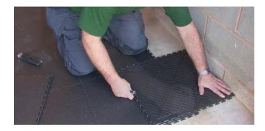
7. Where cuts need to be made, turn the tile upside down and push against the wall. Slide it slightly to one side to reveal the cut marker on the tile underneath.
