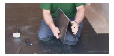
10. Score the tile several times with a concave blade. After a while you should be able to pick it up and bend it back and forth until it snaps.
