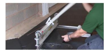
11. Alternatively, you can use a guillotine to make cuts. Once they are cut, they should fit perfectly, leaving a 5mm expansion gap between the tile and the wall.
