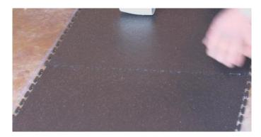
4. The joints of the first tile should meet up with the chalk line.
