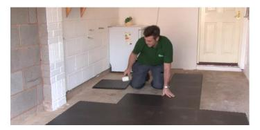
6. Install tiles in incremental steps and work around the centre in a circle to fill the remaining space.
