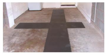
5. Lay the tiles along the chalk line, making sure they are aligned. This way, the tiles should remain straight throughout installation.
