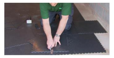
9. Use an upside down tile as a cutting mat. Lay the tile down, and align a metal rule with the marks you previously made.
