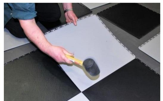
**WHERE TO START:** The starting point for the open joint, the E500/7 & E500/10 tiles, should always be as close to the centre of the room as possible. The hidden joint tile, E500/6, should start from one corner of the room.
