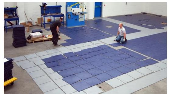
Don't force the tiles, offer up the corner of the tile and gently hammer the joints together.
