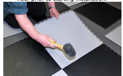
Pic 5. Dont force the tiles, offer up the corner of the tile and gently hammer the joints together.
