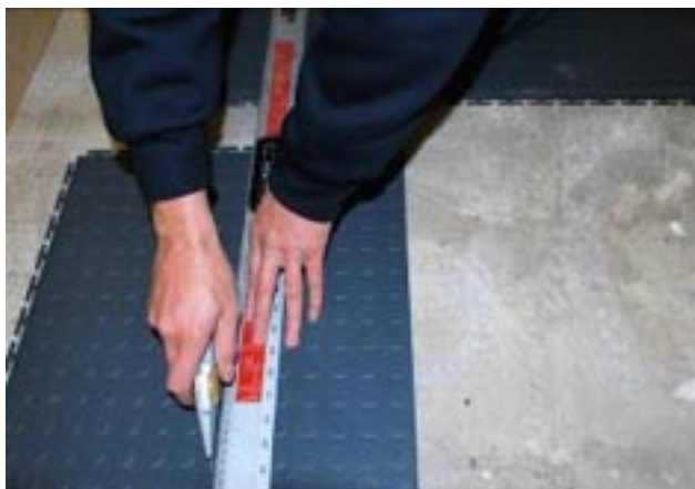
Pic. 2 – Cutting the tiles using our Magnum shear
