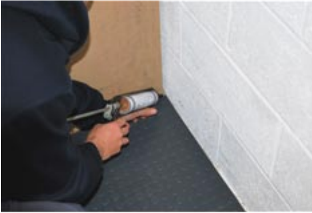
Pic. 4 – Finish around the edges using either a mastic bead or our ecotile sit on skirting
