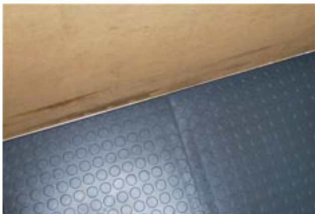
Pic. 3 – Ensure a 5mm gap is left between the tiles and any fixed point
